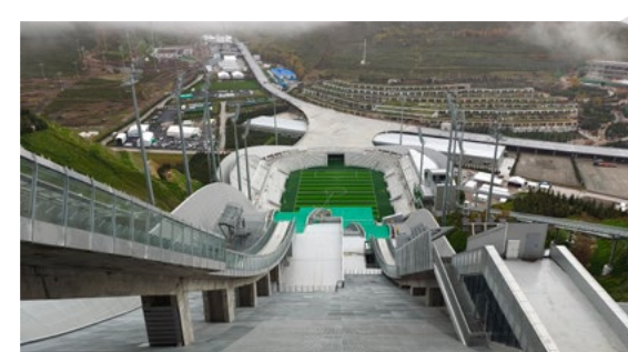
China Building Materials Academy (CBMA) ensures safety for Winter Olympics with environmental governance technology
