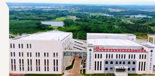
Project of co-disposal of 500t/d domestic waste using cement kilns of Jiangsu Hantian Cement Co., Ltd.
