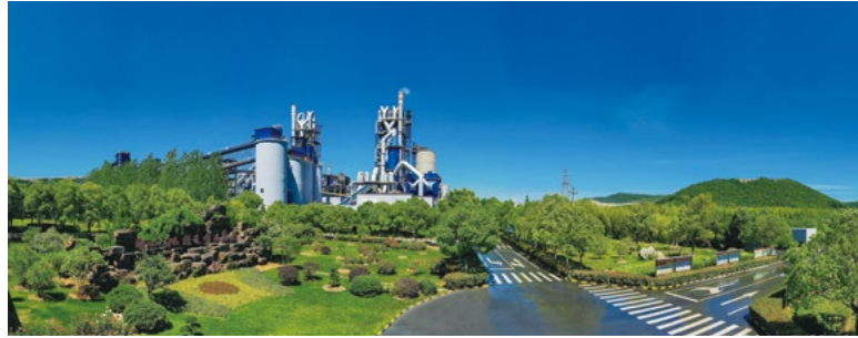
▼ Huaikan Nanfang Intelligent Cement Factory
