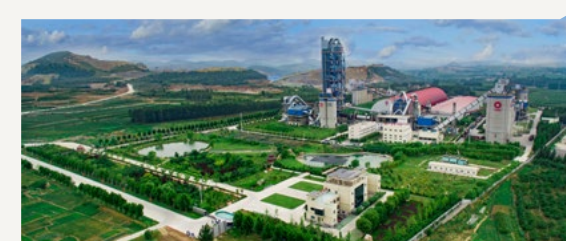
A panoramic view of Green Intelligent Factory of China United Cement Tai'an
