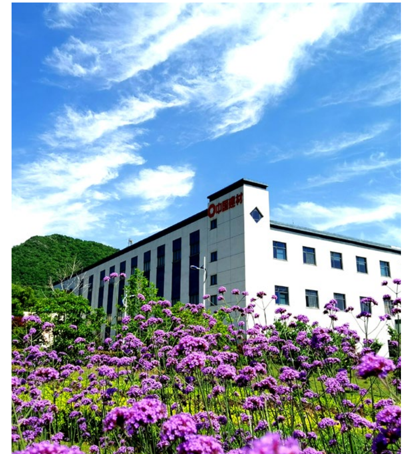
Production Workshop for Co-disposal of Domestic Waste in Cement Kilns of Sinoma Anhui
