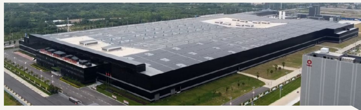
10MW thin-film BIPV application demonstration project - Chengdu 8.5-generation TFT-LCD ultra-thin float glass substrate production line
