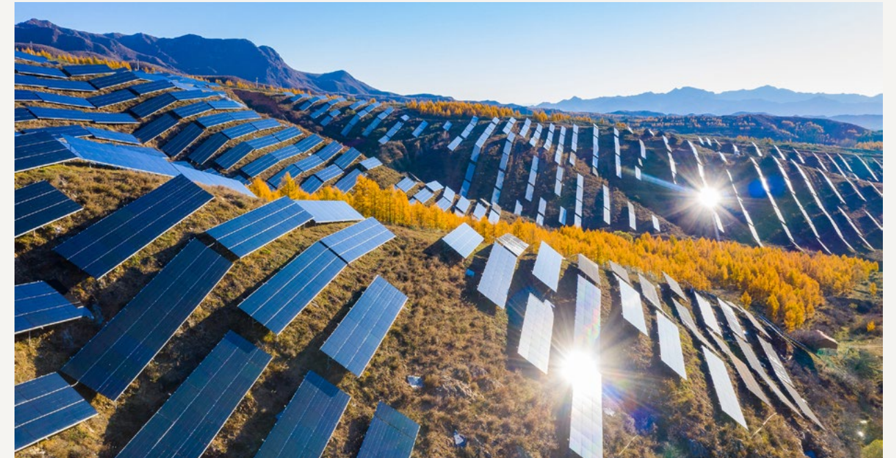
China's first large-scale CdTe power generation glass ground power station -- large-scale mountain restoration power station project in Chicheng County, Zhangjiakou
